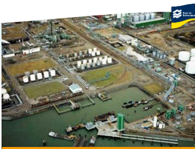
ABENGOA, NEW BIO-ETHANOL PLANT (2010)
