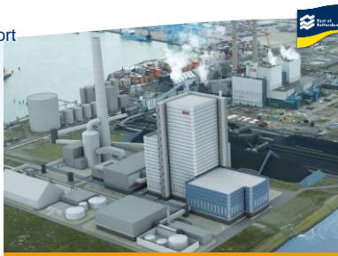
E.On POWERPLANT EXPANSION PROJECT
